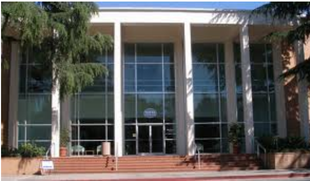
Figure 6-1 SRI International Front Entrance
