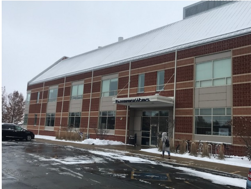
Figure 5-7 Exterior View of the EnvironmentWorks Building Photos
